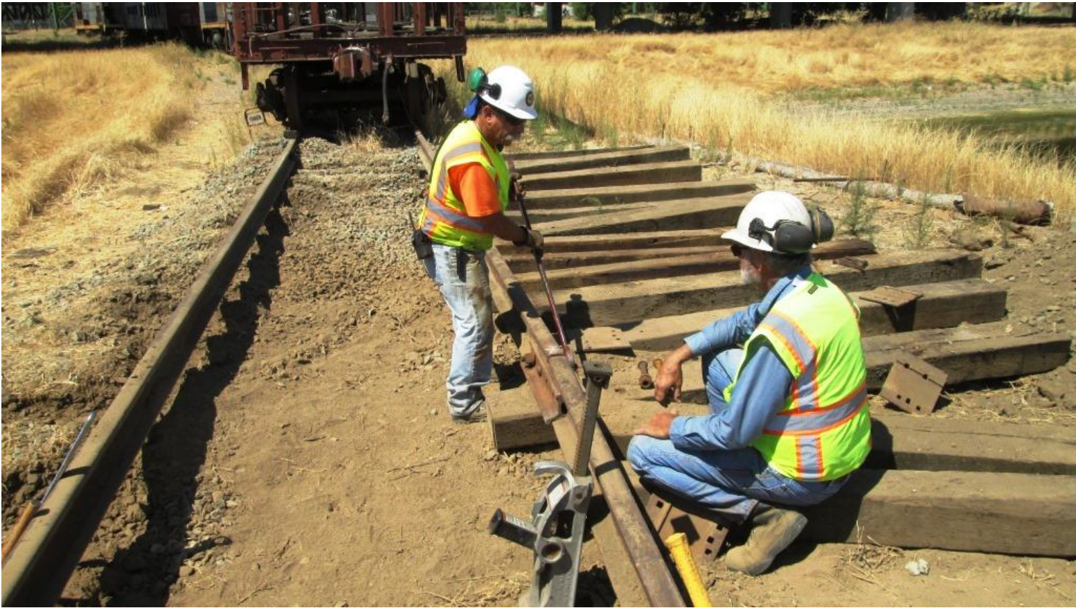
Joe and Alan attempt to bolt the two tracks together. But the gap is too wide
