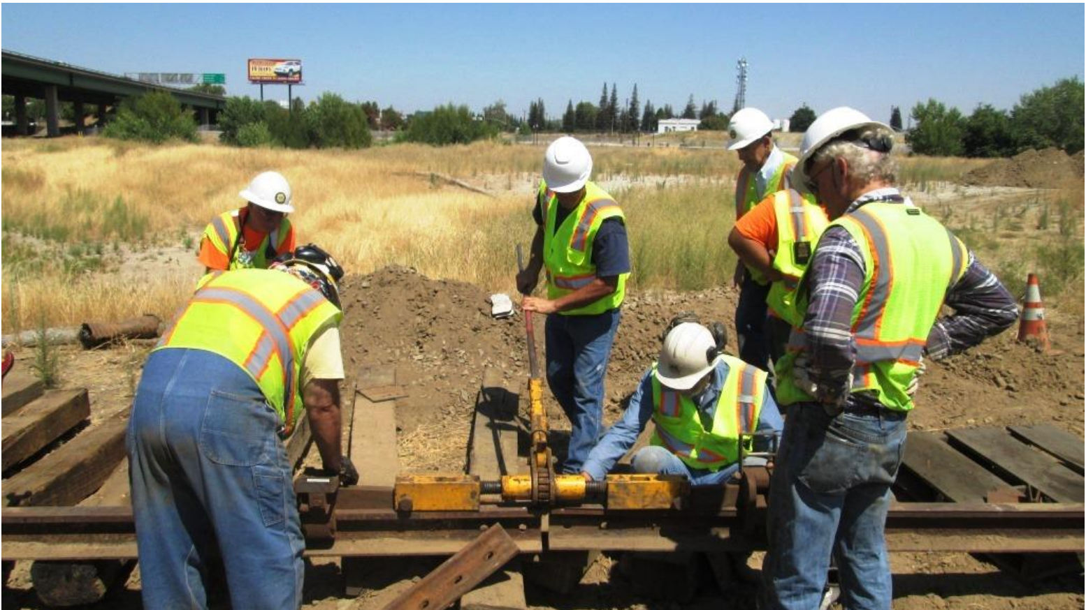
With the rail-puller set up, Andrew starts cranking to close the gap
