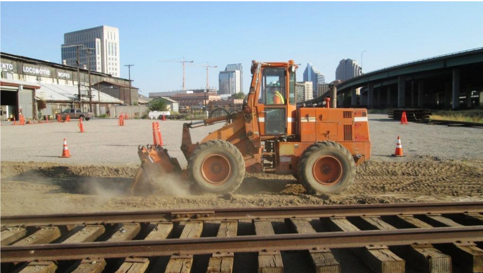
Joe in the loader works to widen the roadbed
