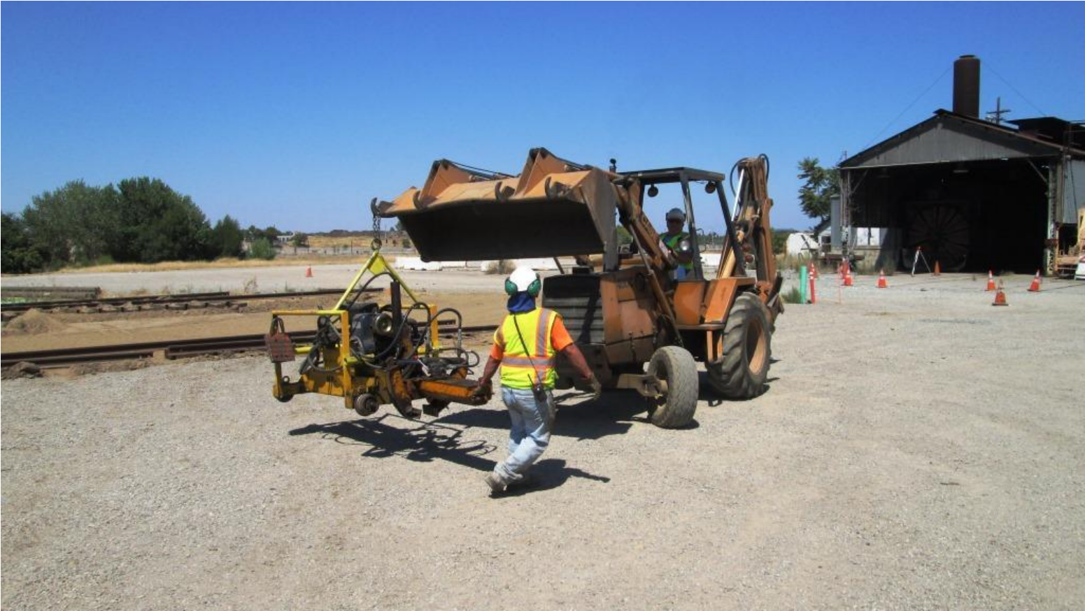
Time to put our toys away... Harry carries the section-gang machine back to the Shops as Joe its from swinging as the back-hoe turns
