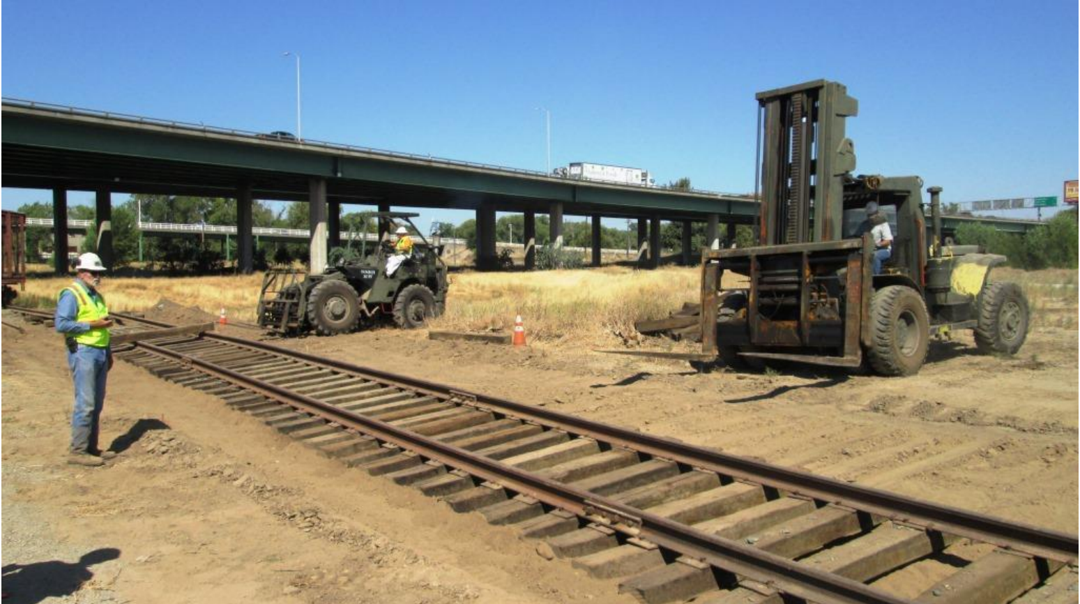
With Big Green and Simba in place, Alan prepare to conduct the movement of the track
