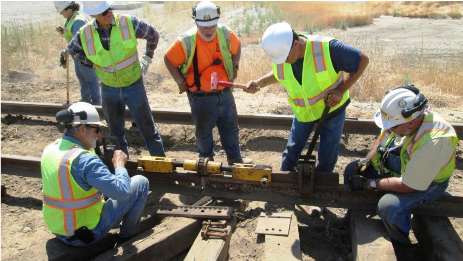
Andrew taps one of the wedges under the rail-clam with the whacker-tool
