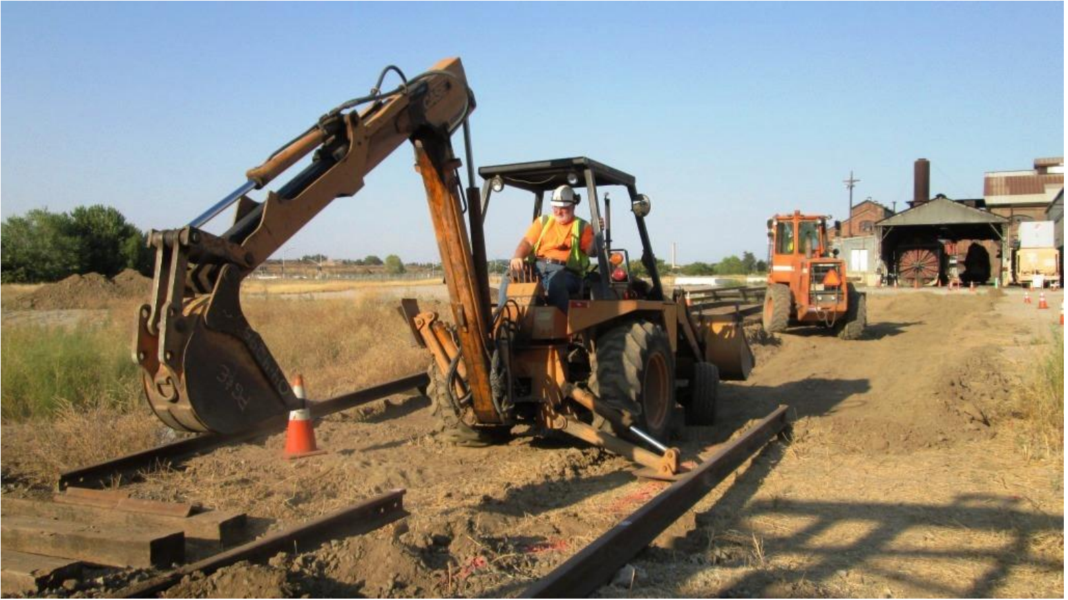
Frank in the back-hoe digs-out the area between the rails as Joe in the loader cuts away more of the roadbed
