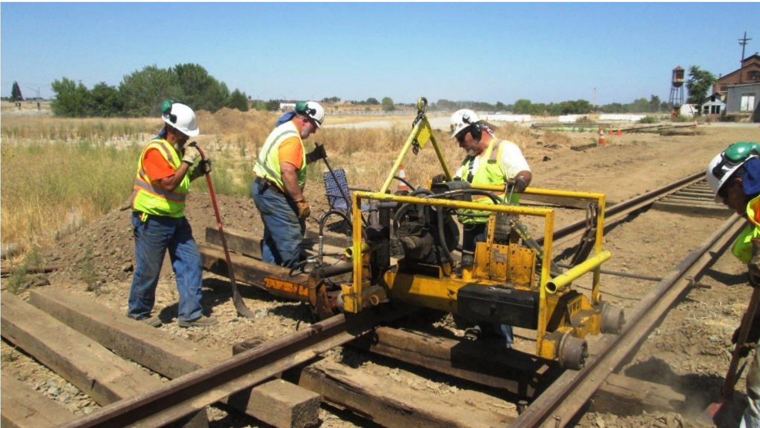
With the section-gang machine working – sort-of, Ed, Frank, and Mike F. start inserting ties
