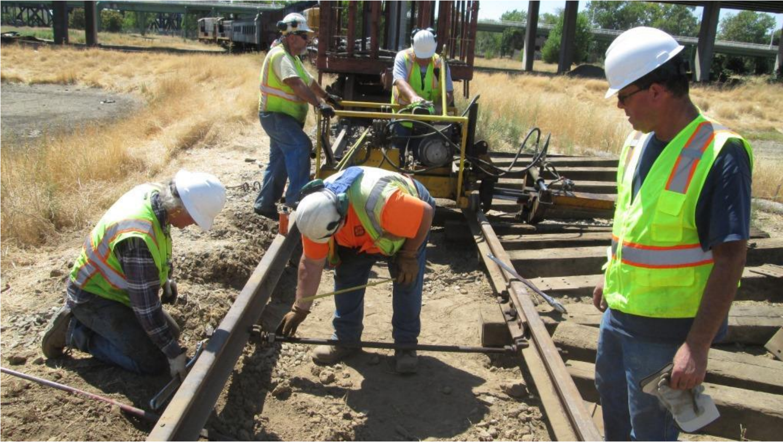
Frank measures gauge as Steve adjusts the gauge-rod. Mike F. and Harry try to get the section-gang machine to work
