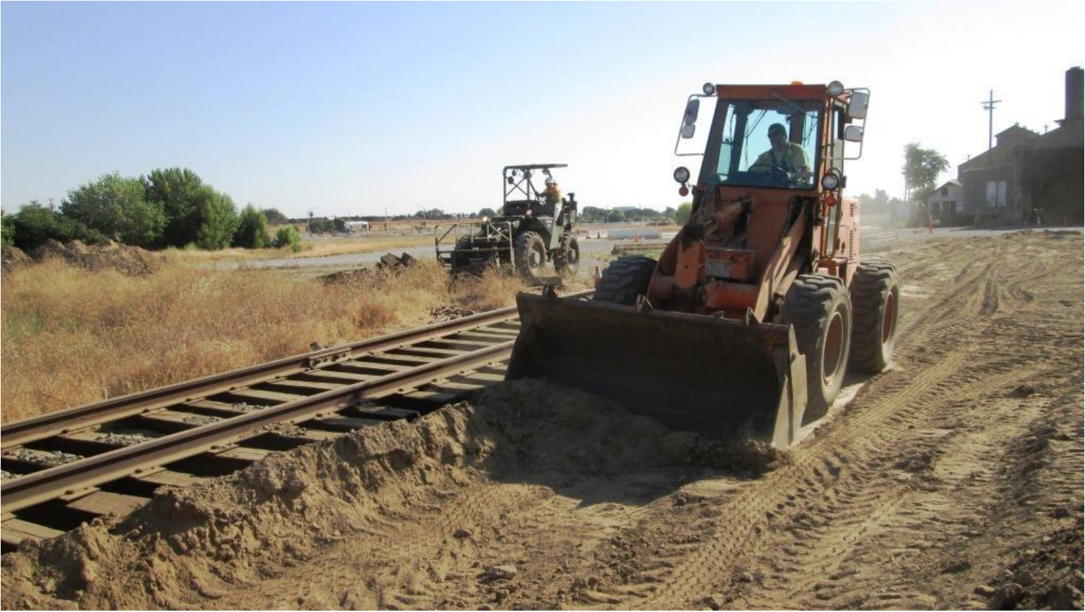
Mike H. on Big Green picks-up some ties while Mike F. in the loader cuts away the dirt berm beside the track
