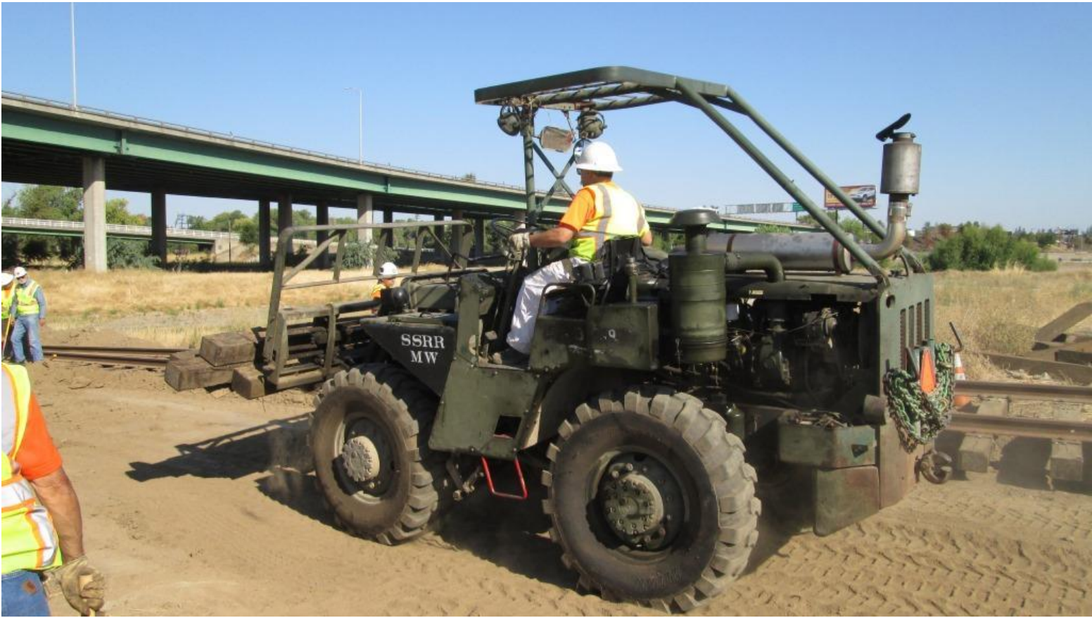
Mike H. brings over some more ties for insertion
