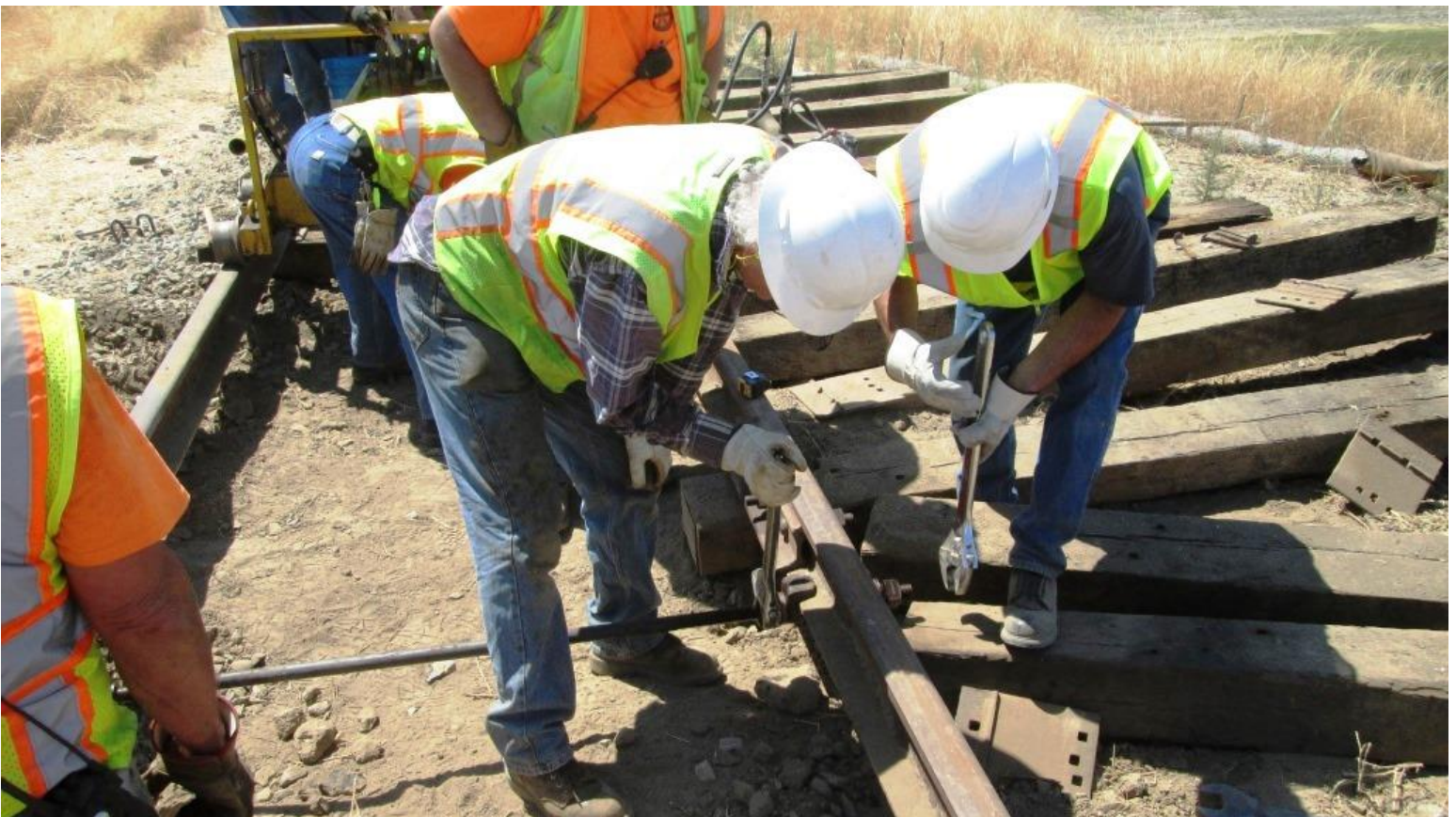
Steve and Andrew tighten-down the rail-clamp on the gauge-rod
