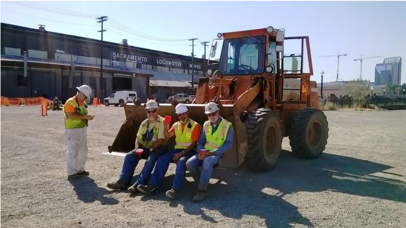
Break time. The loader serves a dual purpose as a bench...
