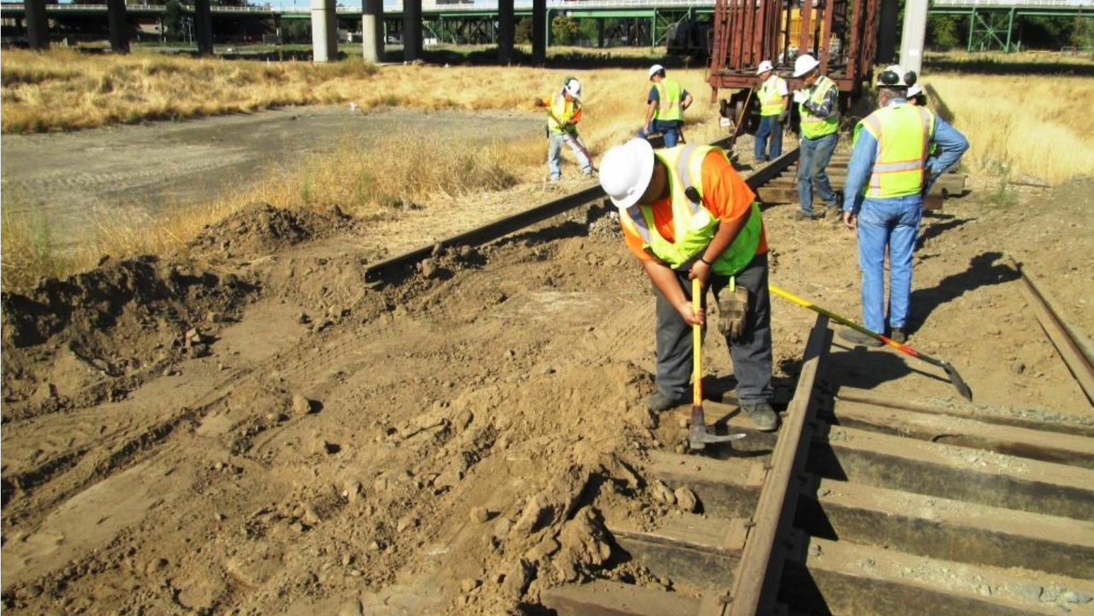
Anthony removes dirt along the tie-ends
