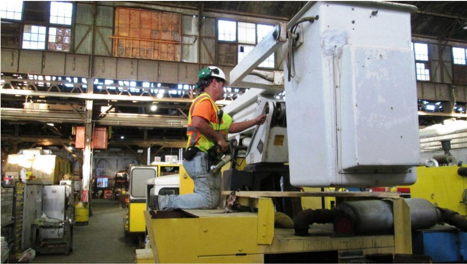
Joe gets right to work servicing the man-lift
