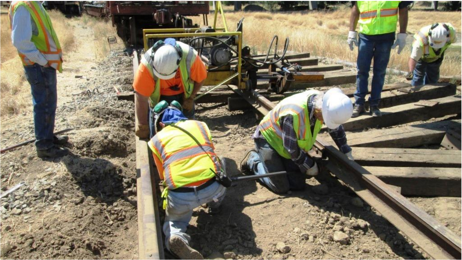
Joe, Frank, and Steve install a gauge rod
