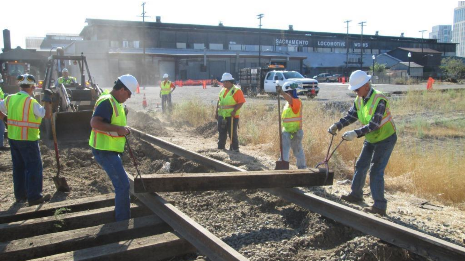
Andrew and Steve slide a tie along the rails while Harry V. uses the back-hoe to level the ground
