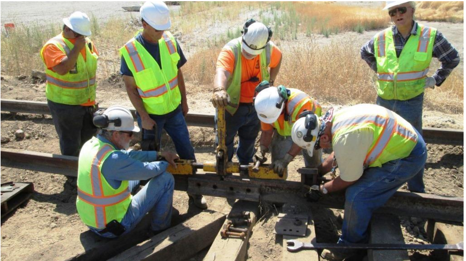
So, the rail-puller is set up
