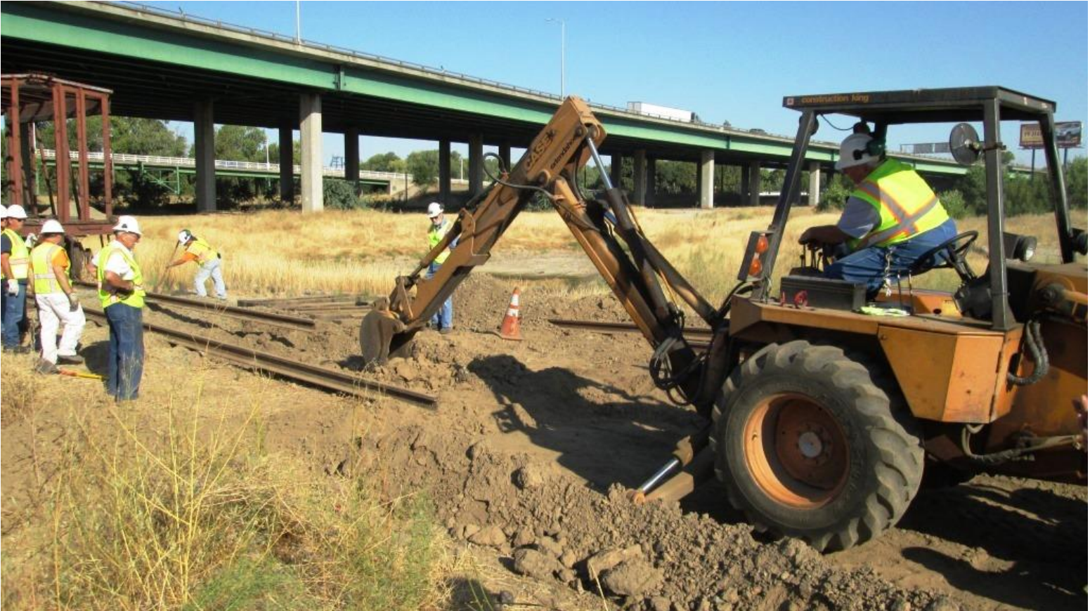
Harry V. on the back-hoe clears out more of the roadbed
